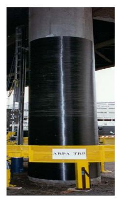
Figure  $10^{18}$  Carbon fiber jacketing of a bridge column.
