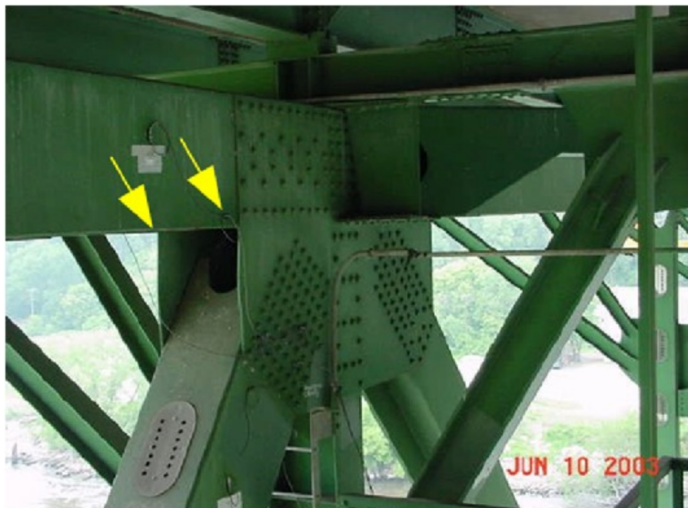
Figure 1: Bowed gusset plates observed at the U10W joint on the actual bridge [2]
